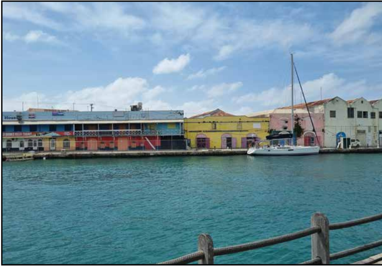
Fig. 1 Desolate and abandoned waterfront cafes and an empty carenage (picture by De Waal, February 8, 2024).
