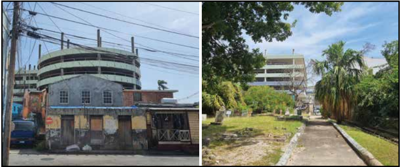
Fig. 4 Left: The City Central Mall car park towering over the traditional buildings in Suttle Street (seen from Reed Street, looking south). Right: The City Central Mall car park, dominating the view from St Mary's Church towards the east (pictures by De Waal, February 8, 2024).
